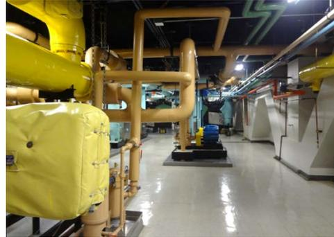
The building also effectively uses the residual energy in its steam condensate. Instead of discarding all of the steam condensate generated in the building, it is used to pre-heat their closed loop circulating hot water system. This strategy saves money and energy by reducing the amount of steam needed to heat the circulating loop, resulting in lower steam bills.
